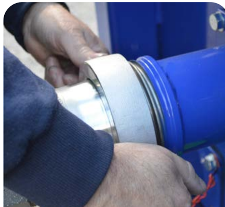
Ball valve being installed on the top outlet.
