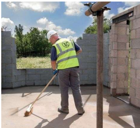
1. Clear debris from work area
