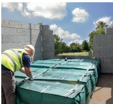
7. Continue to assemble until the floor area is covered
