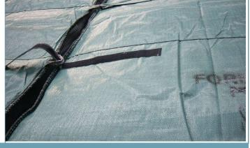
3. Connect bags together by pulling velcro straps through loops on adjacent bag or by attaching plastic connectors.
