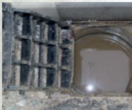
Prevents pollutants entering a watercourse e.g., silt, heavy metals, hydrocarbons and suspended solids.
