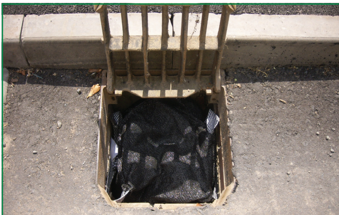
5. Close gully grid.
