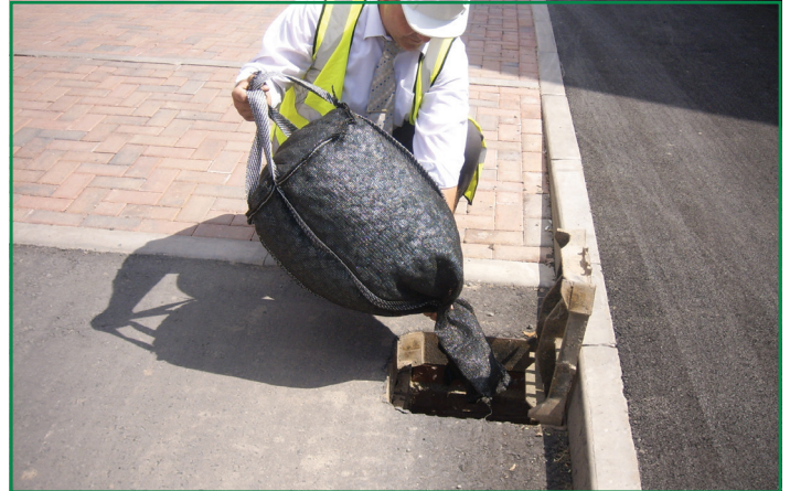
2. Hold handles at top of the Gully Guard, work beads to top and insert base into water filled gully pot.
