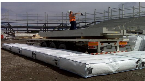
7) Ensure entire perimeter of vehicle/structure is completely protected by bags. Installation to be checked by competent person.
