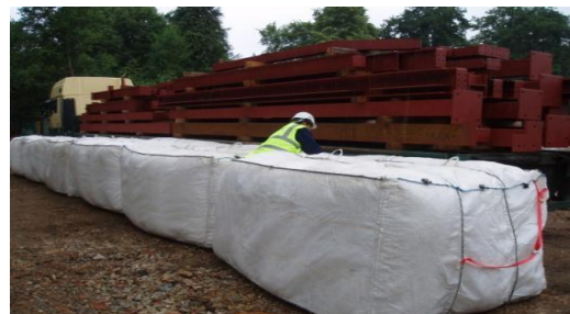
7) Ensure entire perimeter of vehicle/structure is completely protected by bags. Installation to be checked by competent person.
