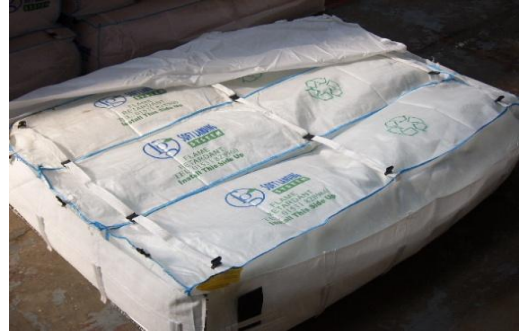
2) Place 3 no. Standard Soft Landing bags (for a 600mm high Wallet or 6 bags per 1200mm high bag)
