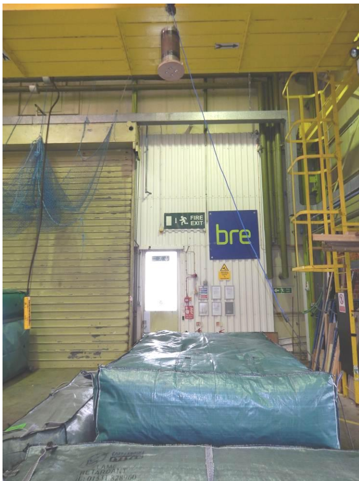
Figure 1 View of the double stack of 600mm Lorry bags
