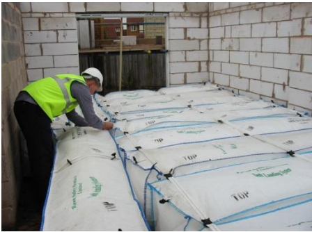
5) Continue to assemble until the floor area is covered.
