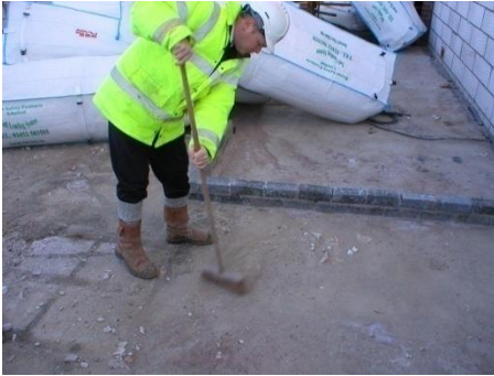
1) Clear debris from work area.
